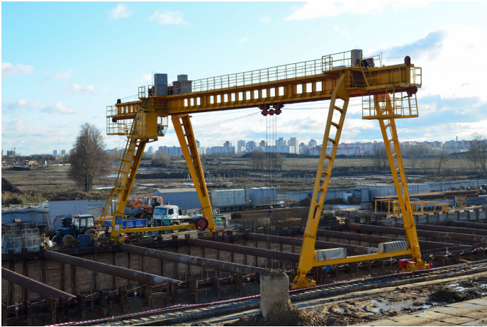
Gantry crane at a construction site
